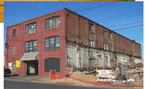
Demolition of adjacent structure
