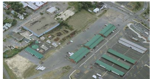
Aerial view – After
