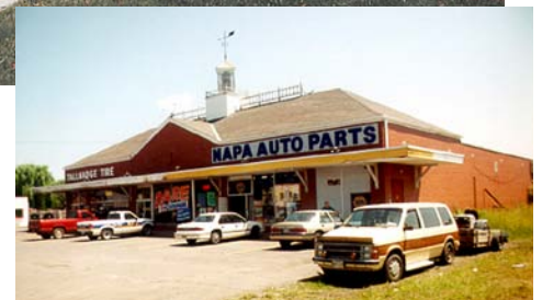
Site prior to renovations
