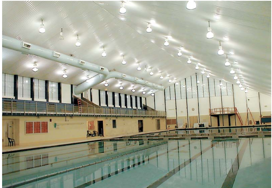
View of new roof and interior restoration
