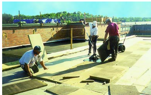
Construction in progress
