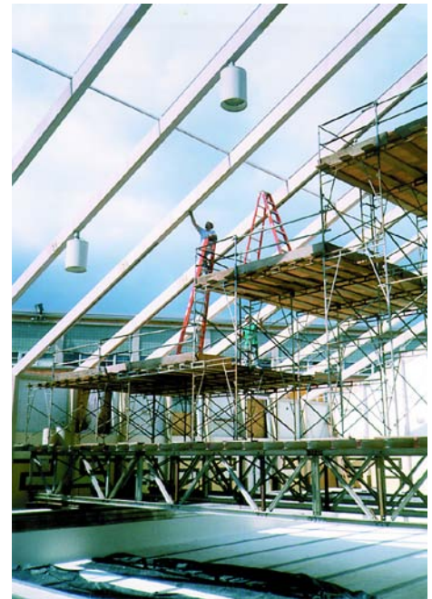
Scaffolding erected over pool for construction
