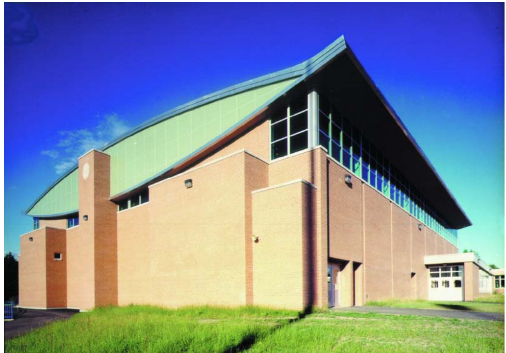
Exterior view of gymnasium and upsweeping truss system
