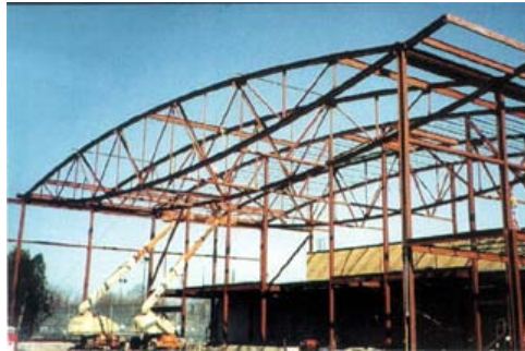
Steel truss erection
