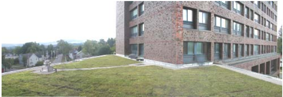
View of Green Roof Connector
